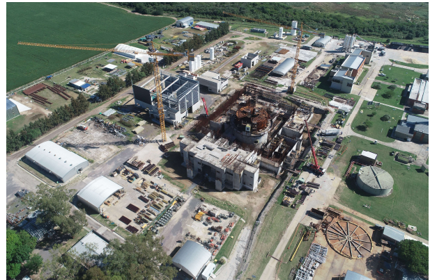
CAREM25 construction site
