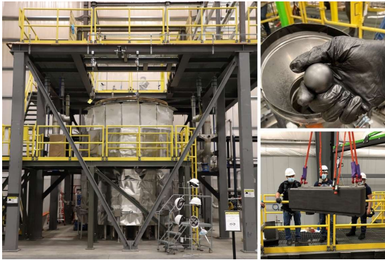
Engineering Test Unit under construction
