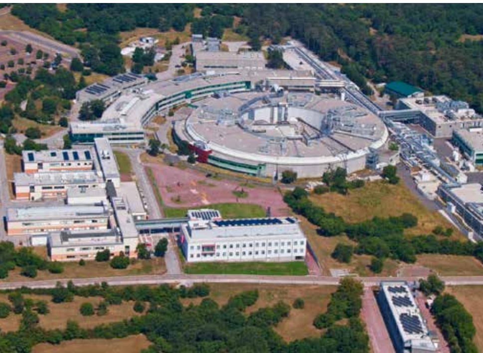
Elettra-Sincrotrone Trieste in Italy.
