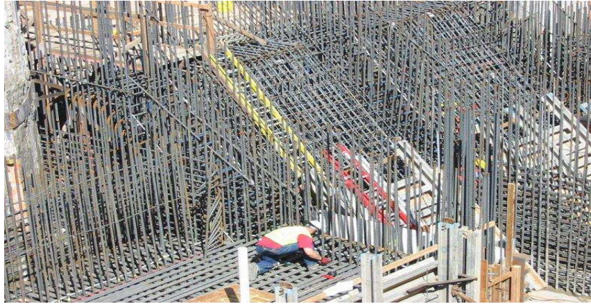
Figure 21. Steel plate reinforced concrete and slip-forming.
