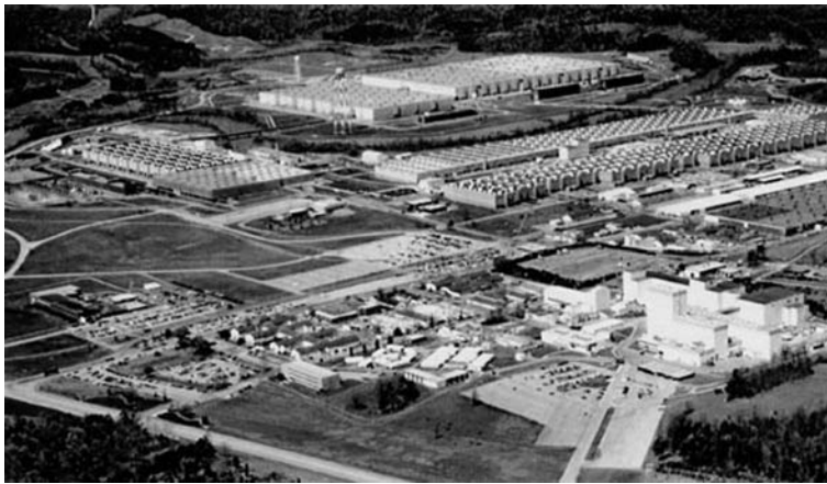
FIGURE 9.2 Oak Ridge Gaseous Diffusion Plant in Oak Ridge, Tennessee.
