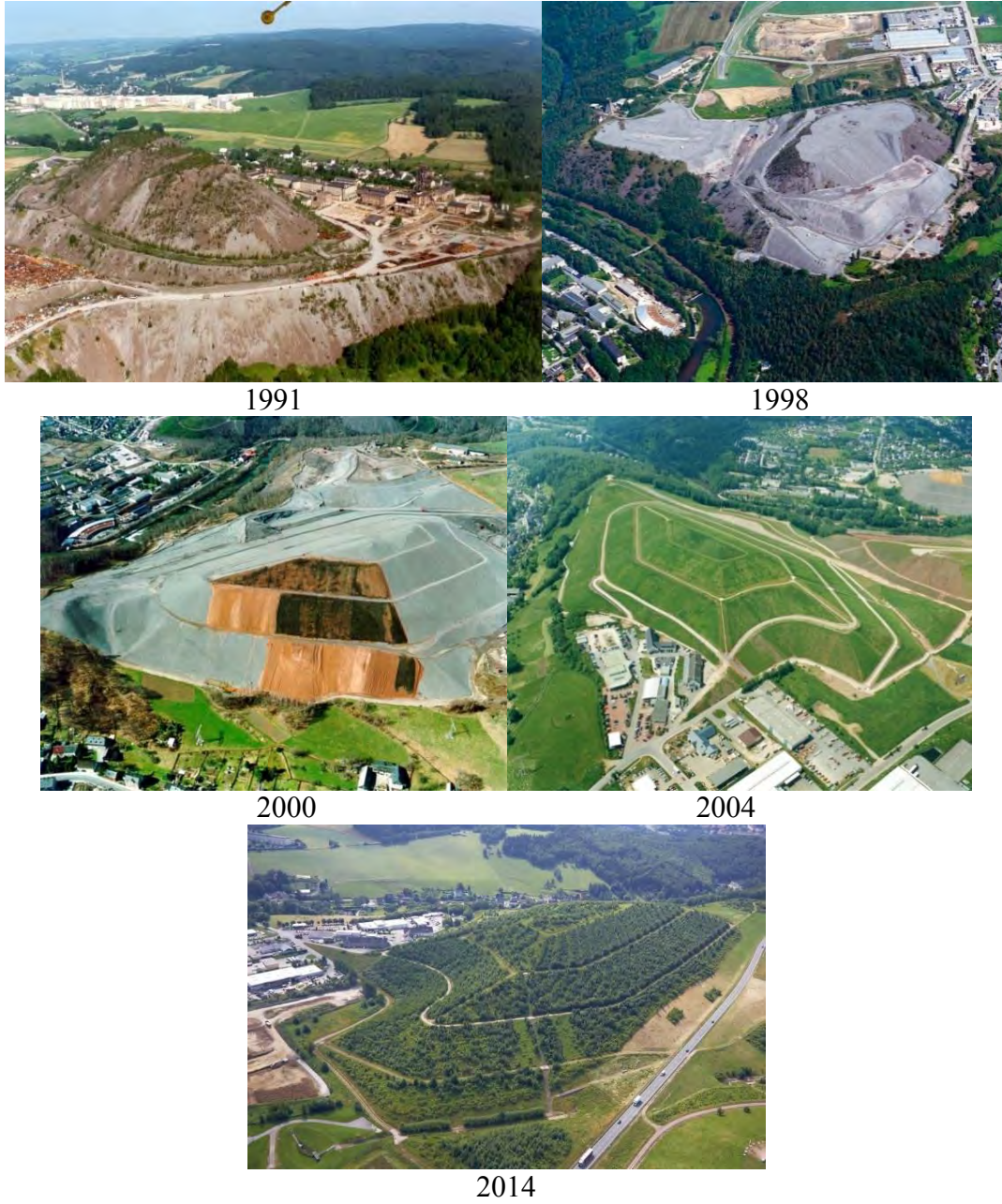
FIG. 4. Coverage of waste piles in Schlema-Alberoda (Aue site).
