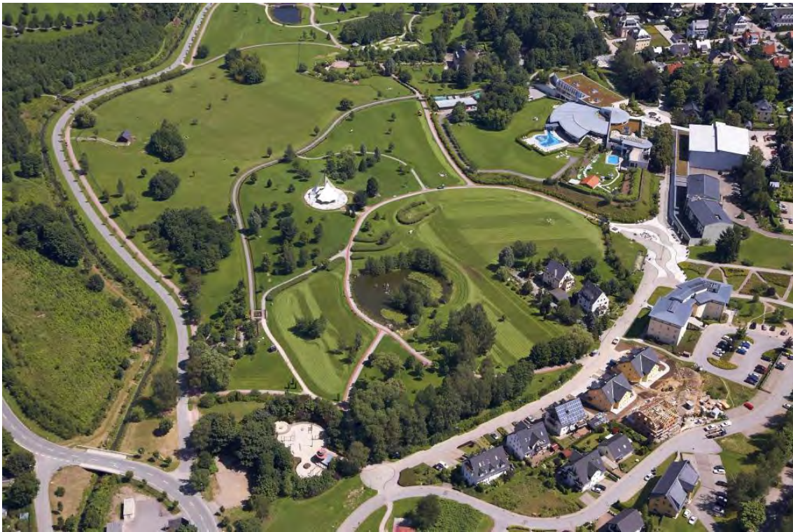
FIG. 7. Aerial view towards the Schlema spa garden, with reshaped, covered, and recultivated waste rock piles on the left.
