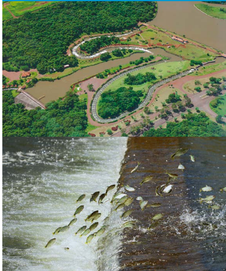
An aerial view of the fish ladder at the Itaipu hydropower plant. Local fish, known as lambari, swim up the ladder's steps (Eletrobras).
