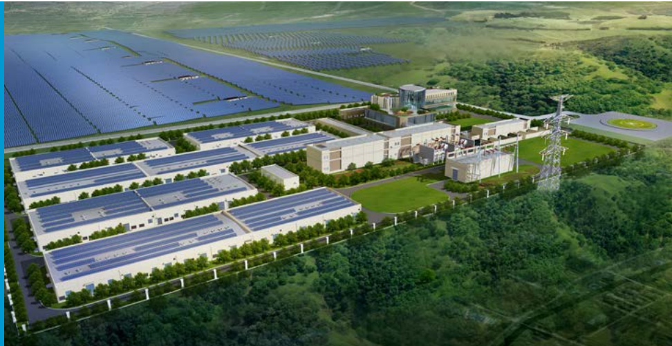
The Zhangbei National Demonstration Project in China combines 140 MW of wind and solar generation, 36 MWh of energy storage and a smart power transmission system relieving intermittency challenges (SGCC).
