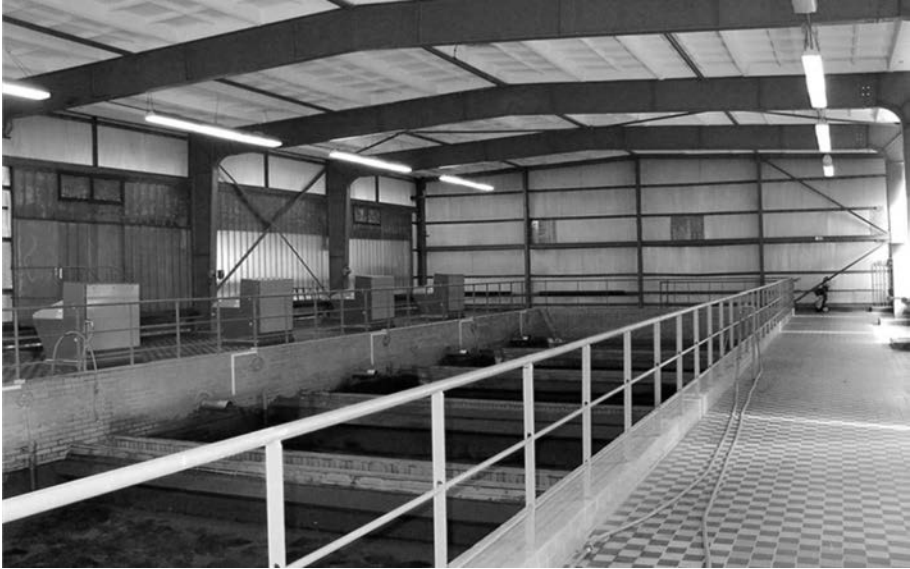
FIG. 1. The filtration hall with open filters.
