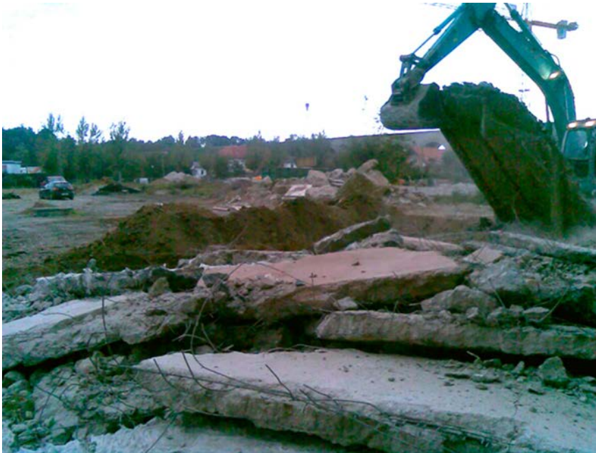
FIG. 3. Demolition of the non-contaminated parts of the building.
