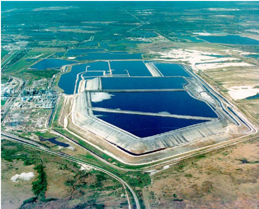
FIG. 3. Process water retained in a phosphogypsum stack.
