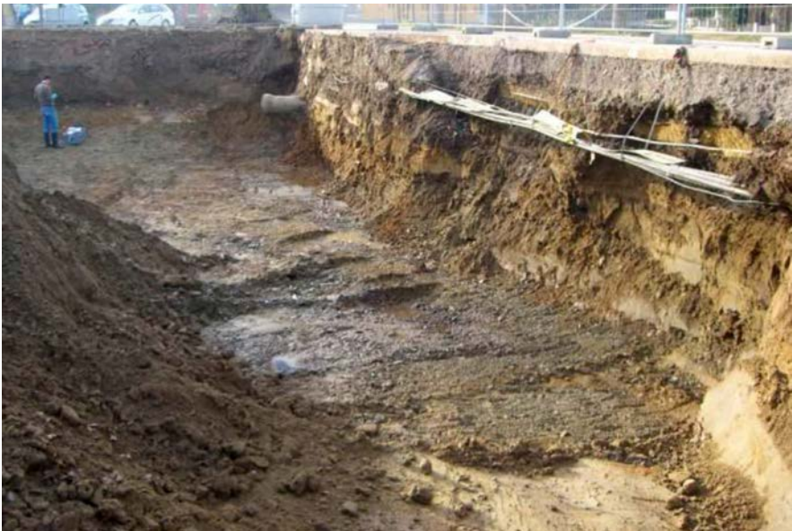
FIG. 8. The excavated pit during final inspection.
