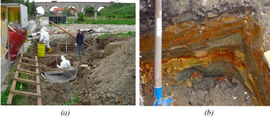
FIG. 7. The excavation work: (a) early stages and (b) highly contaminated zone.
