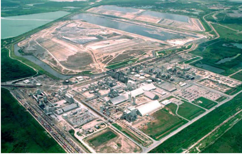
FIG. 2. Phosphoric acid production facility and phosphogypsum stacks.
