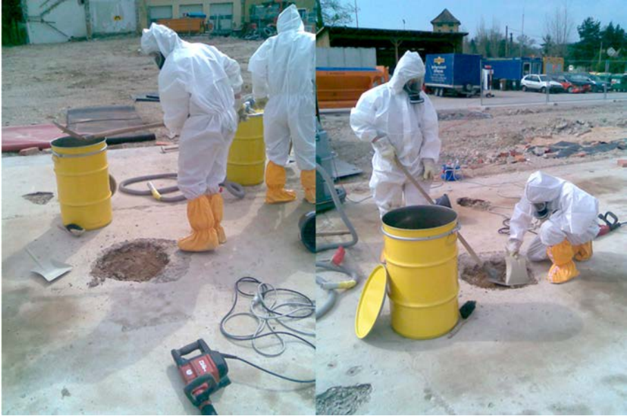
FIG. 5. Remediation of a hotspot.
