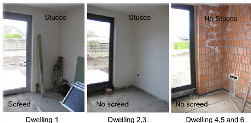
FIG. 3. Various construction stages of the dwellings.
