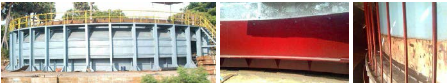
FIG. 9. Mock-up for welding of roof slab hanging shell and main vessel.
