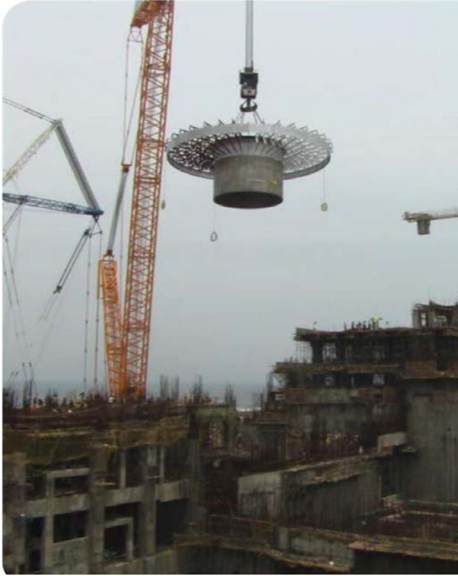
FIG. 8. Safety vessel erection mock-up.
