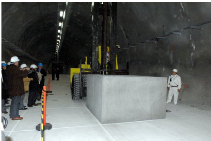
FIG. A-13. Emplacement of the first waste disposal package at the disposal facility in Bataapati, Hungary.
