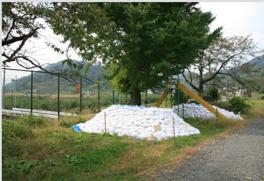
FIG. A-16. Temporary storage of soil removed at a model remediation project at the Tominari elementary school, city of Date, October 2011.
