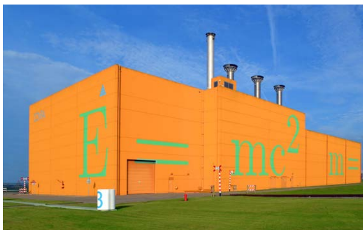
FIG. A-11. HABOG intermediate waste storage facility, The Netherlands.
