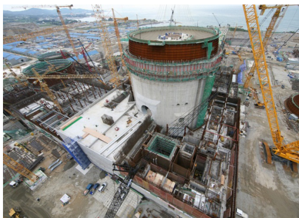
FIG. A-2. Construction at Shin-Kori-3 in the Republic of Korea.
