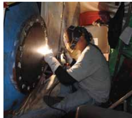
Welding at Watts Bar 2 Steam Generator
