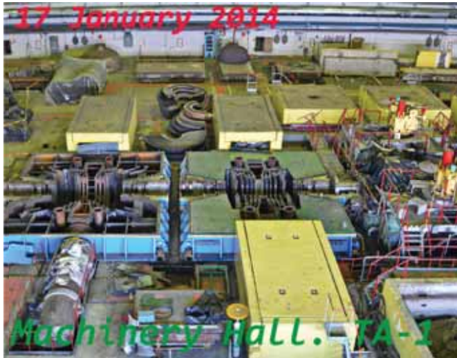
Nuclear Power Plant Ignalina-2 equipment dismantling and decontamination
