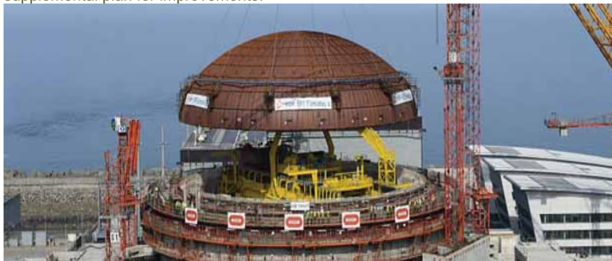
Flammanville - 3 EPR 1600MW (photo Edf)
