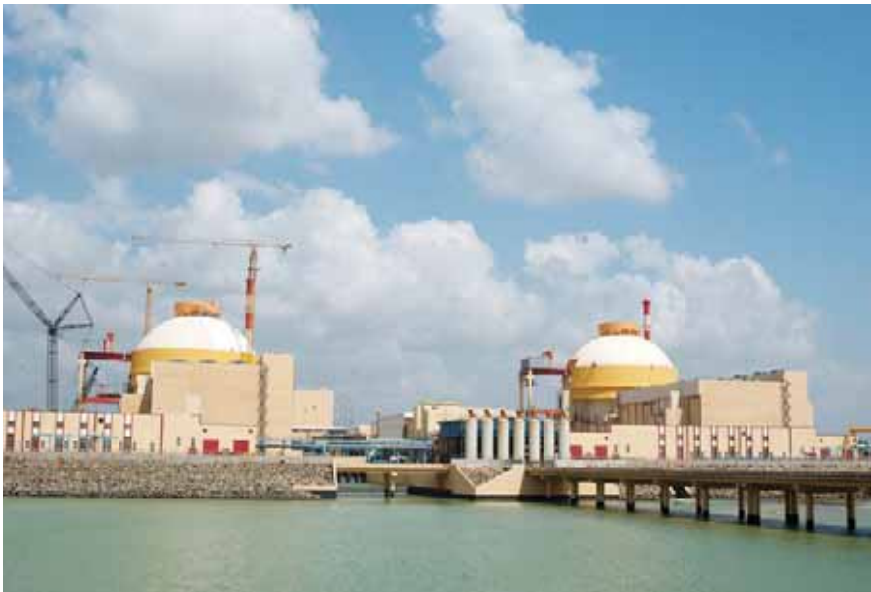
Kudankulam NPP -Two reactors (2x950 MW -VVER) - India. Reactor 1 connected to the grid in October, 2013 (photo: Atomstroyexport)
