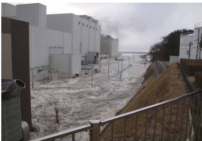
NPP Fukushima-Daiichi after the first wave tsunami
