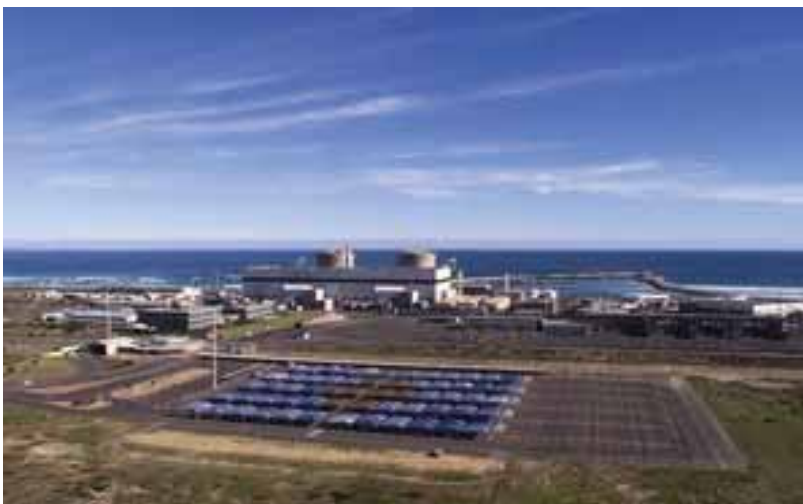
Nuclear Power Station Koeberg (Photo by: Ruvan Boshoff)
