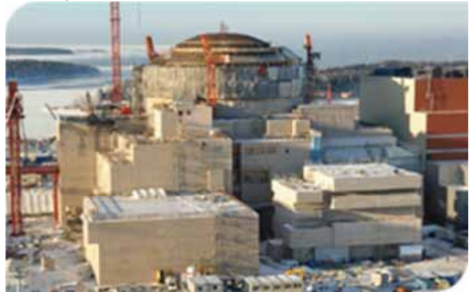
Nuclear Power Plant Olkiluoto 3 (photo AREVA)
