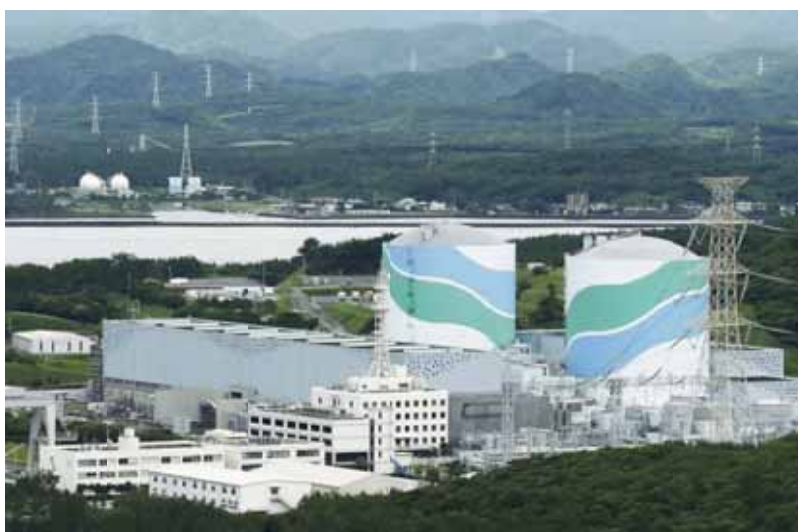
Nuclear Power Plant Sendai 1 and 2
