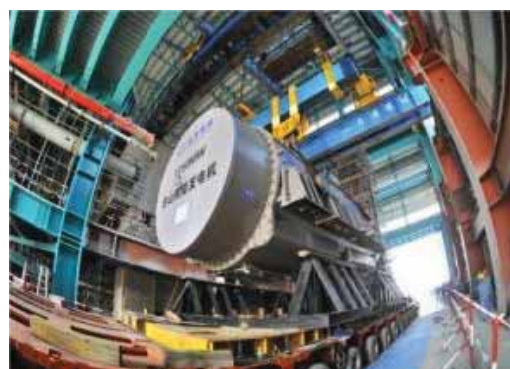
Taishan 1 –EPR 1600 under construction
