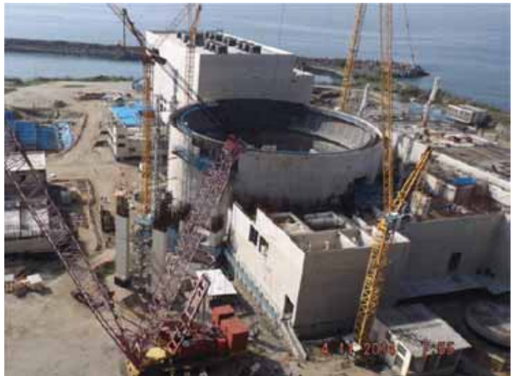
Angra 3 –Reactor Building Status (photo Eletronuclear)
