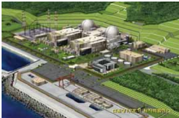
Shin-Kori 1 and 2 - Photo: KHNP (Korea Hidro and Nuclear Power)
