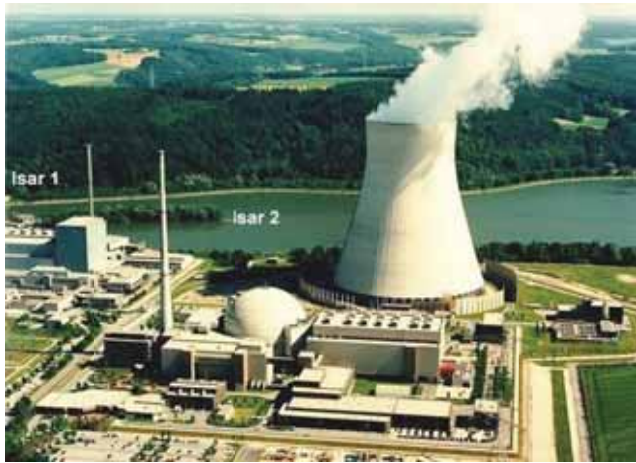
Nuclear Power Plant Isar-2, second biggest nuclear generator in 2010 - closed in 2011
