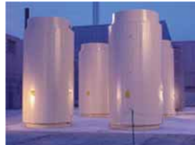
Dry storage Example ( Holtec International Co)
