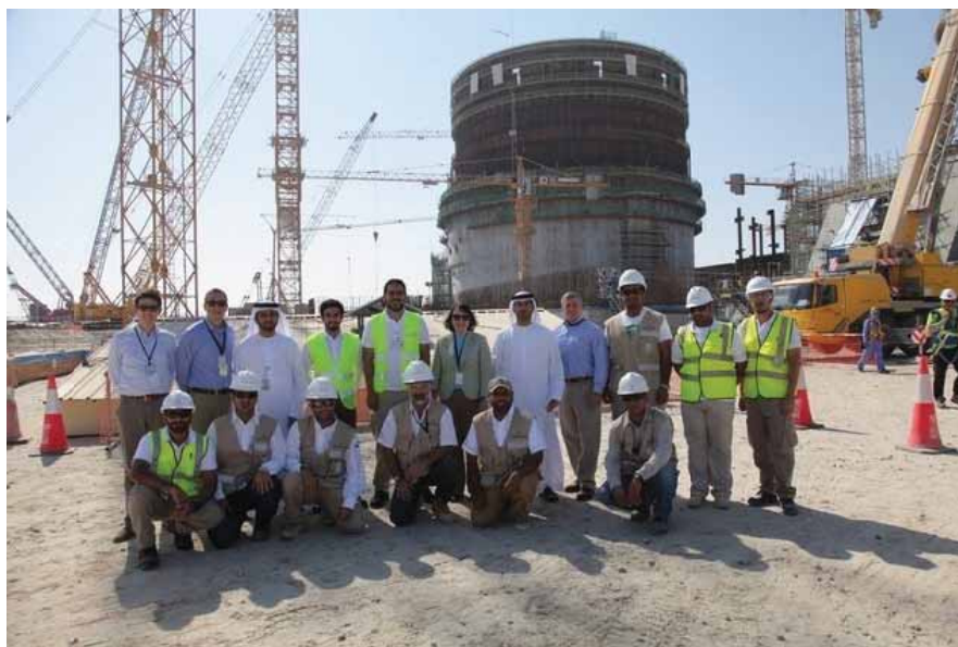
Barakah1 and 2 - Under construction
