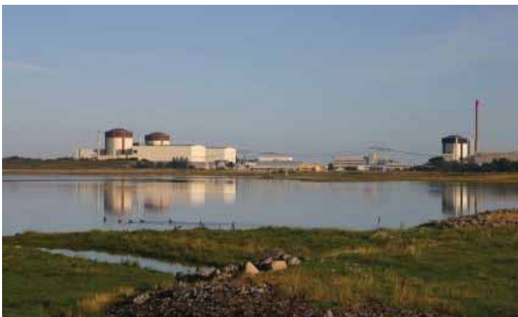
Nuclear Power Station Forsmark
