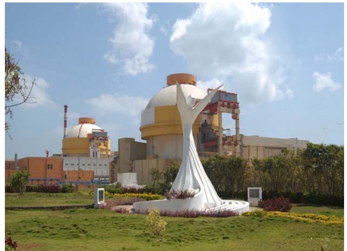
Kudankulam -Two reactors (950 MW-VVER) under construction at India. Reactor 1 was connected to the national grid October 2013 - (Photo: Atomstroyexport)
