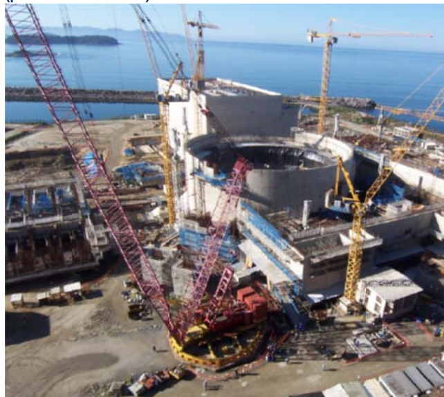
Angra 3 – status of construction (Aug 2013) Reactor Building (photo Eletronuclear)
