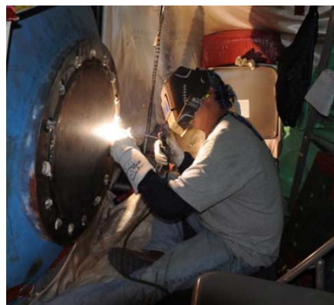
Welding at Watts Bar 2 Steam Generator
