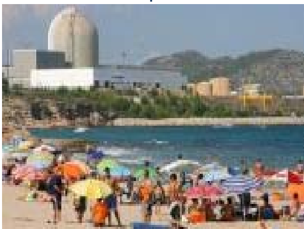
NPP Vandellos 2 – Spain
