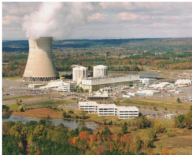
Arkansas Nuclear One Generating Station Courtesy: Entergy Nuclear
