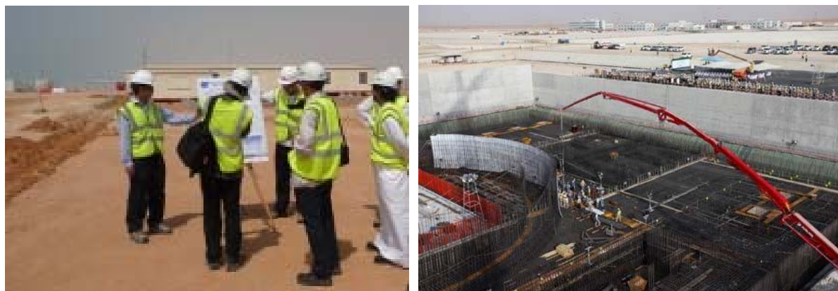
Barakah1 and 2- Under construction
