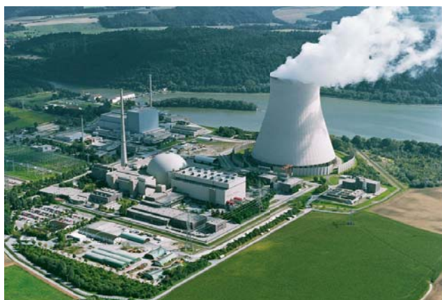
Nuclear Power Plant Isar-2 , second biggest nuclear generator in 2010 – closed in 2011
