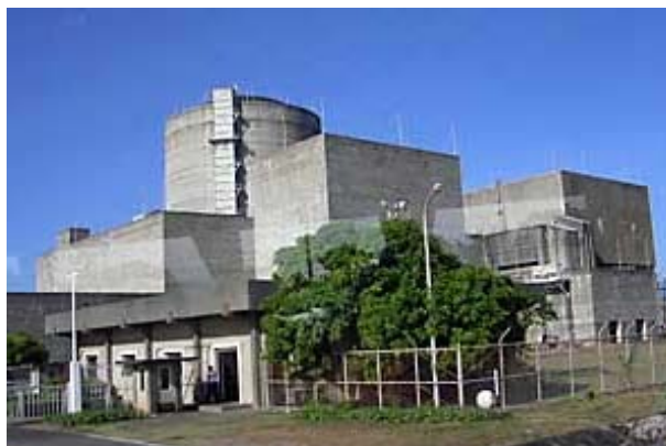
Philippines - Bataan Nuclear Power Plant -photo IAEA Ready – has never operate
