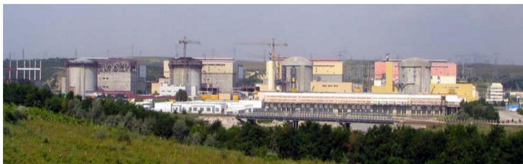
NPP Cernavoda – Romania – The units 1 and 2, on right side are in operation
