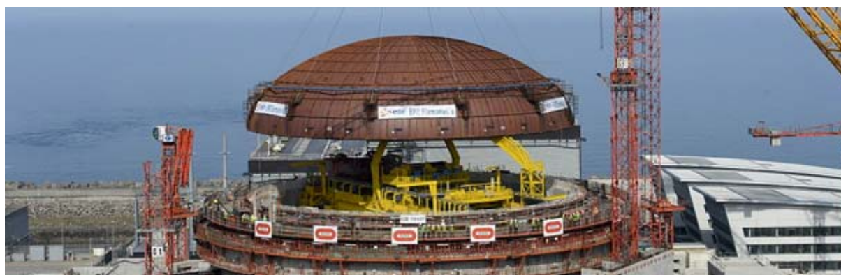
Flammanville - 3 (photo Areva)
