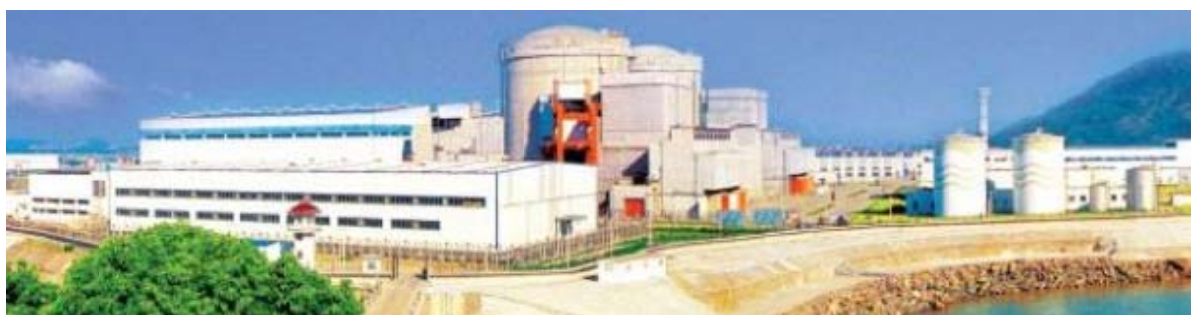
Unit 4 at China's Qinshan Phase II commercial operation
